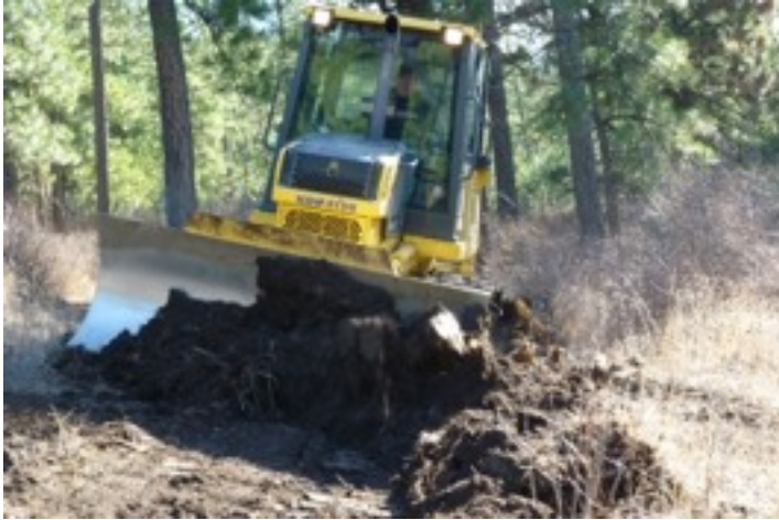
Doug Peery working on a water bar at LLORV cleanup
